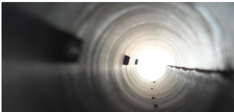
(Picture 1、2 ,section of the pipe hole)
